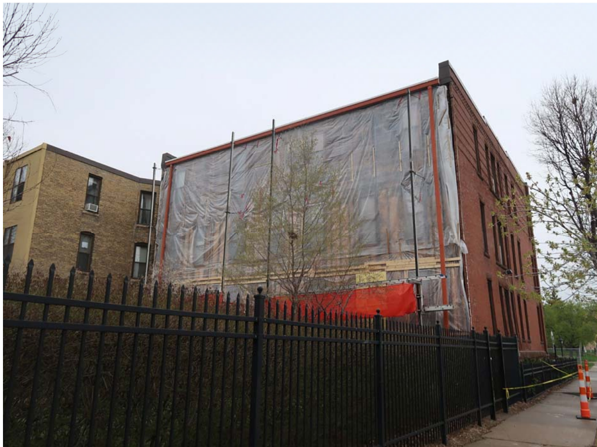
Photo 2 - Rear of the Building
