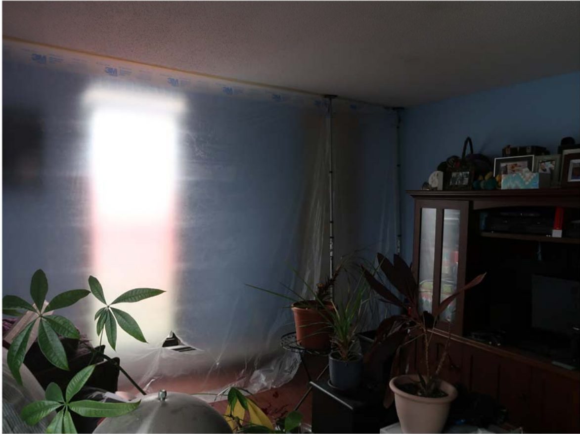
Photo 7 - Unit 5 Exterior Wall Where Window Work Will Be Done
