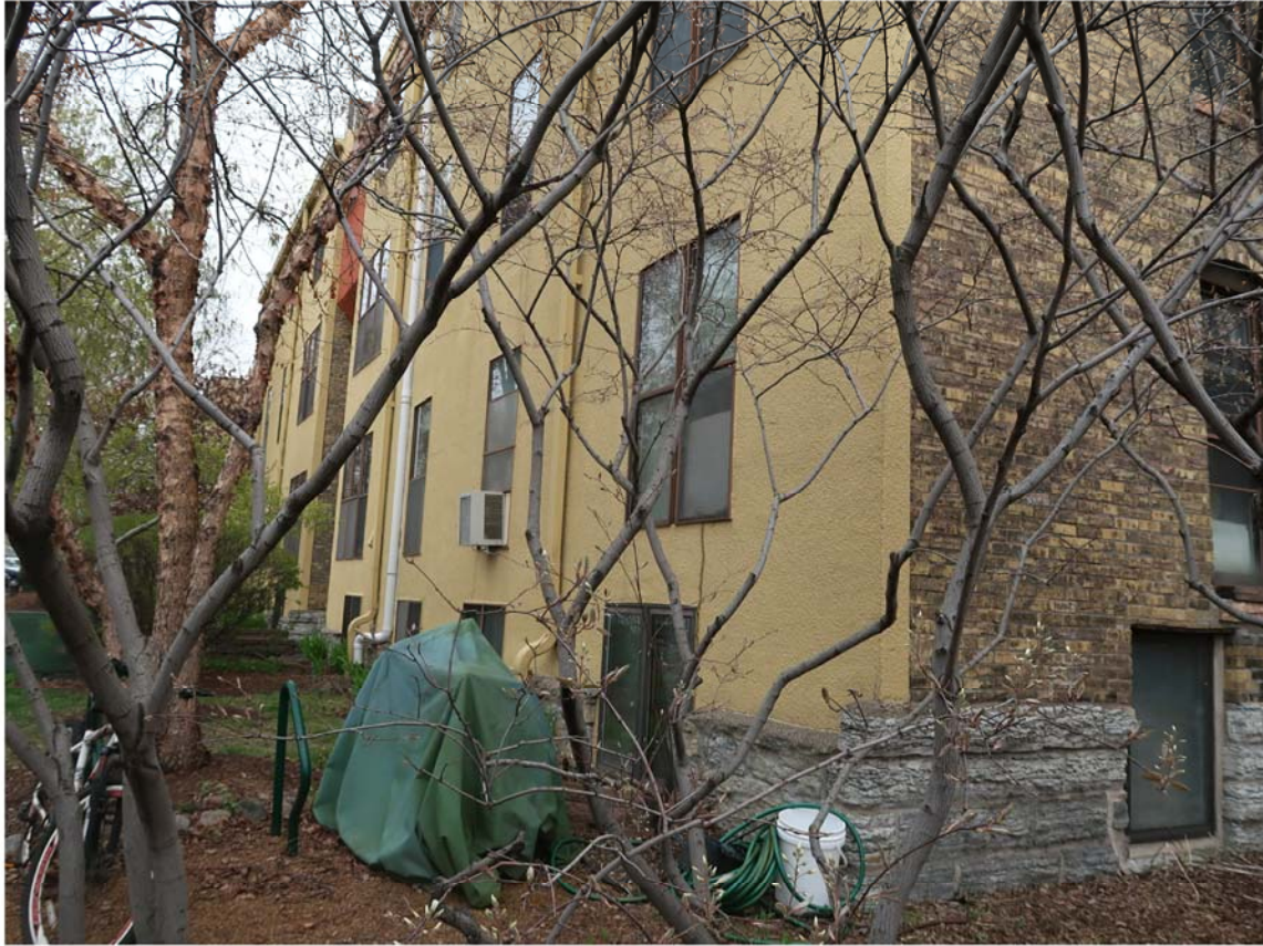
Photo 3 - Stucco Was On the 1801 Building Similar to the Next Door 1809 Bldg
