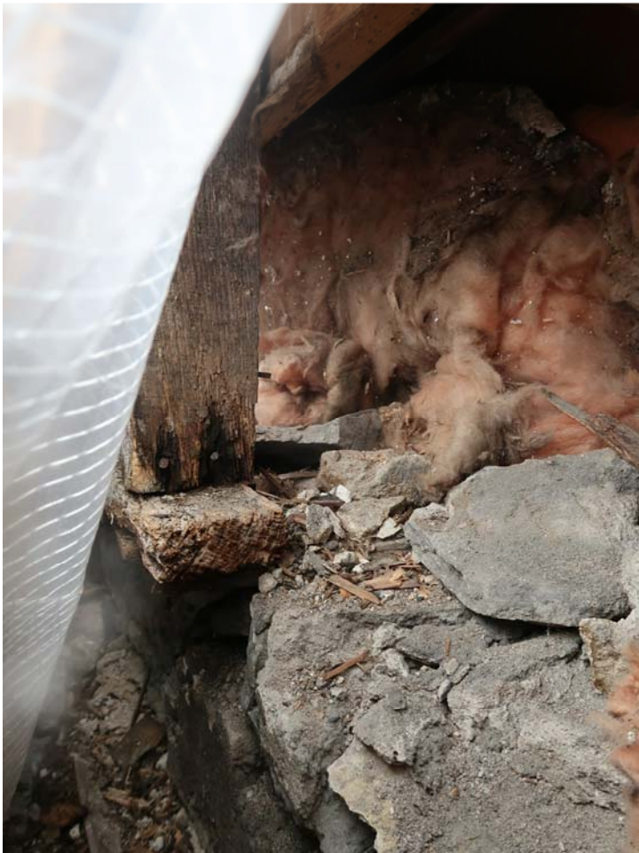
Photo 6 - Looking Inside the Wall Cavity
