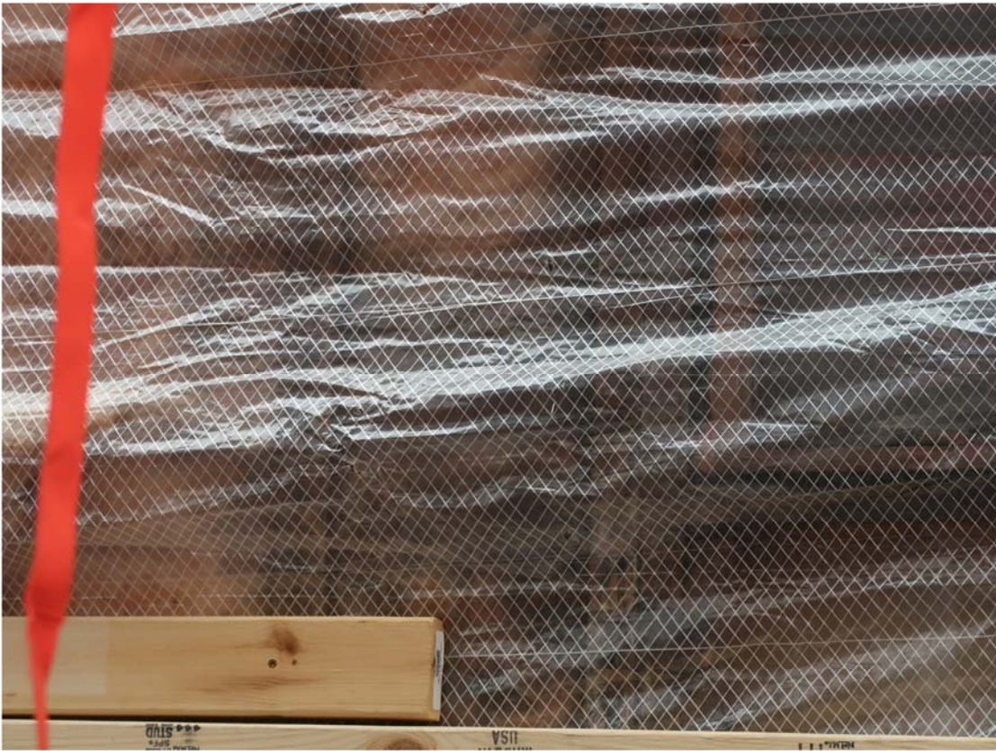
Photo 5 - Close up of Polyethylene Covered Opened Exterior Wall
